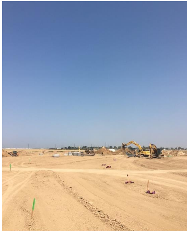
Construction of wet utilities at Sky Ranch
